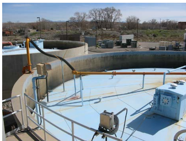
Secondary Digester with Floating Cover
