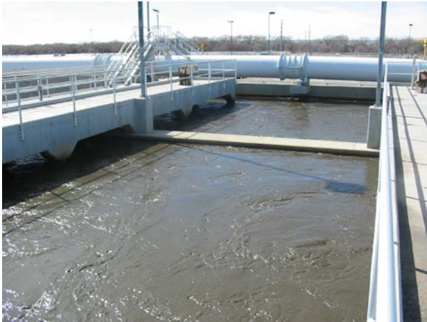
Denitrification Basin Anoxic Stage
