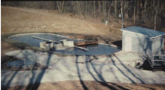
Activated sludge oxidation ditch treatment plant
