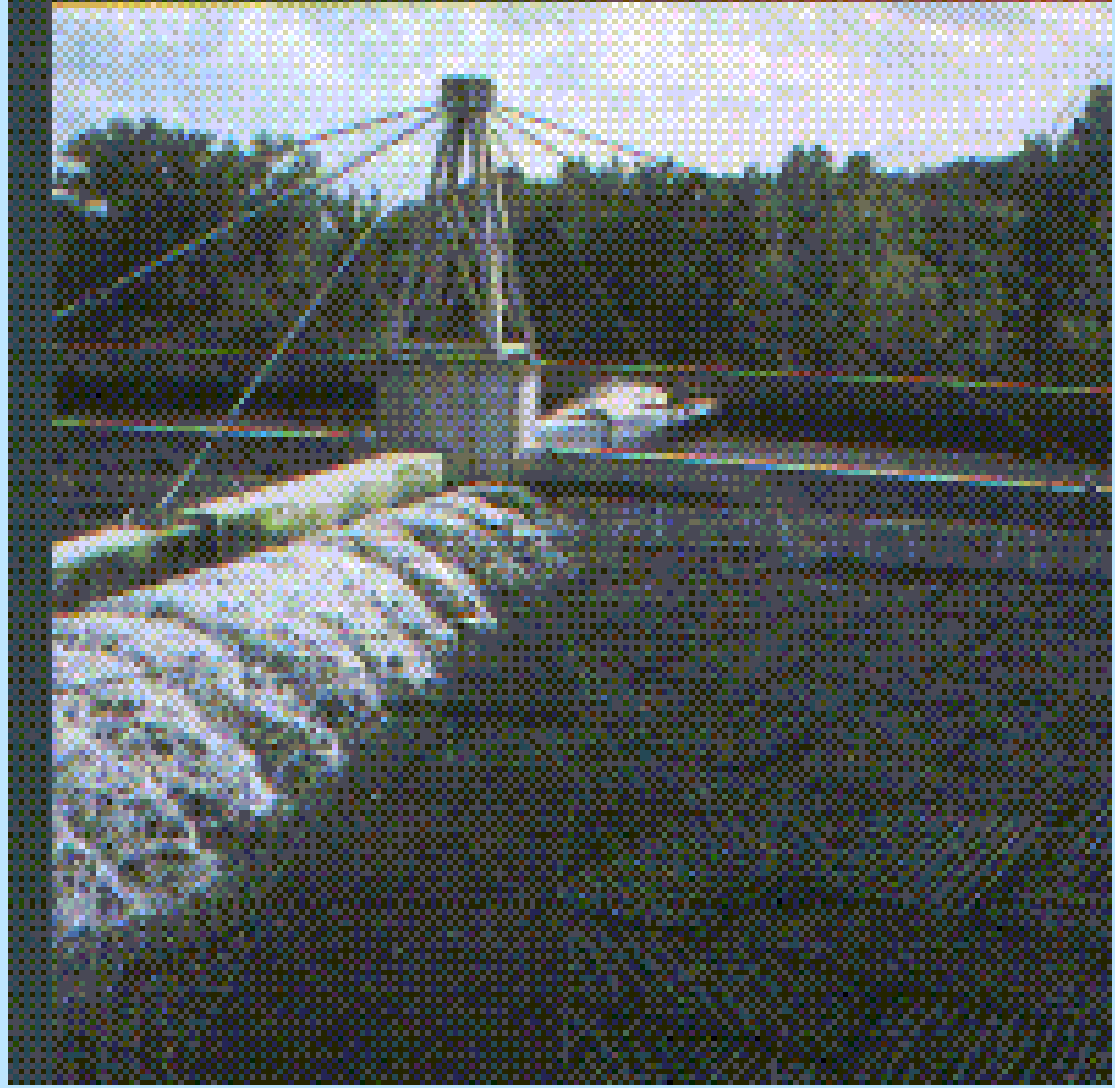
A TRICKLING FILTER
