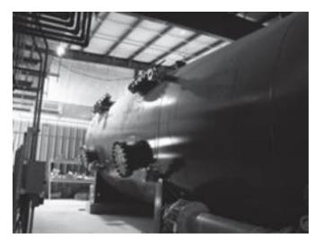
**Figure 15.2 -** Biological Activated Carbon Absorber (S. Hanson photo file)
